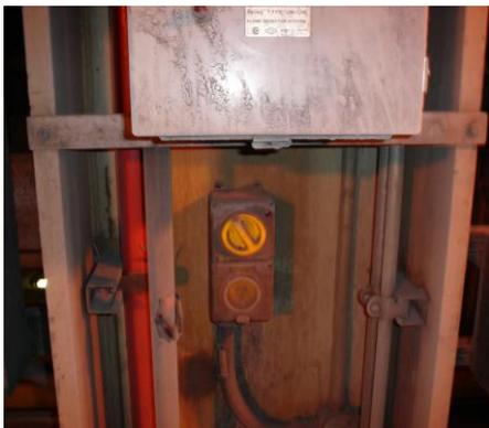
In this case the correct Ex outlets were removed and replaced with standard IP 66 - 3 pin outlets
