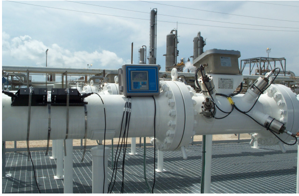
Dual Beam Reflect Mount Installation at Yslosky LA, USA (Line Pressure: 58 barg)
