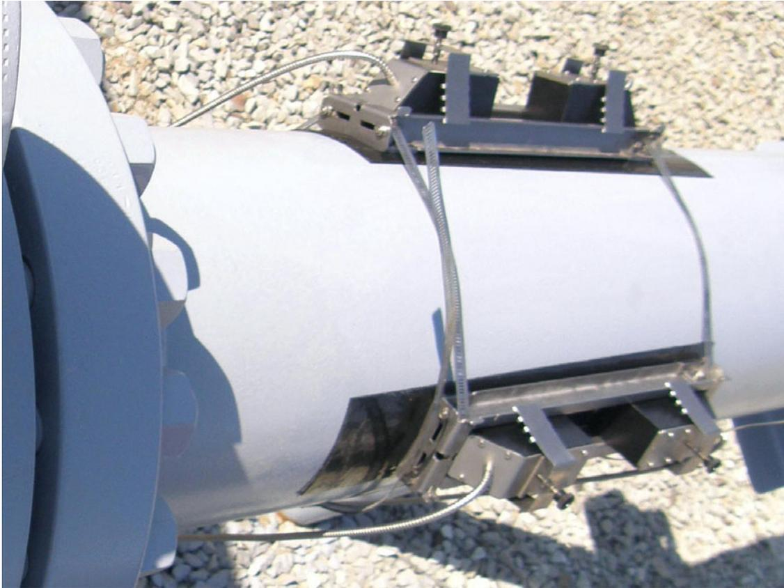
Figure 3. Transducers mounted on pipe in reflect mode.
