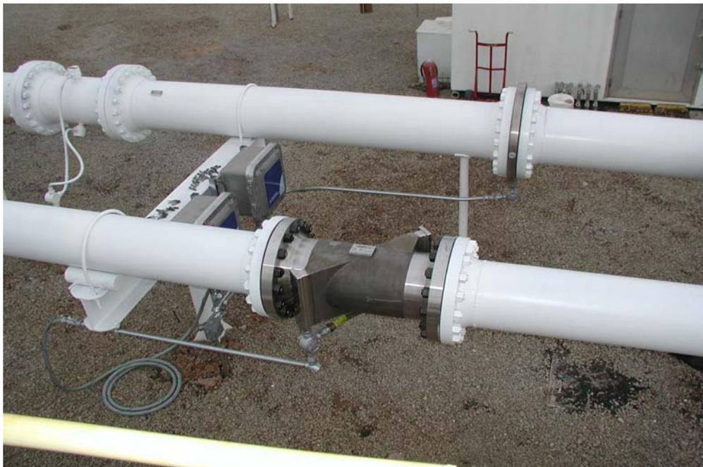
**Figure 2: Installed 4-Path Chordal LFM – 240C**
