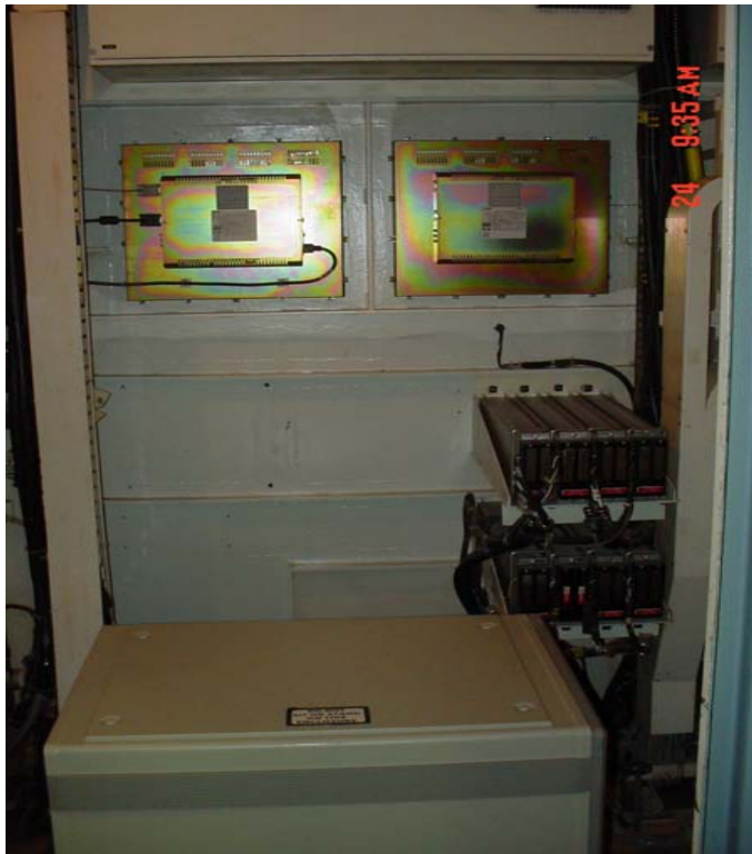
VERTICAL BOARD AFTER RECORDER REMOVAL AND FLAT PANEL HSI INSTALLATION
