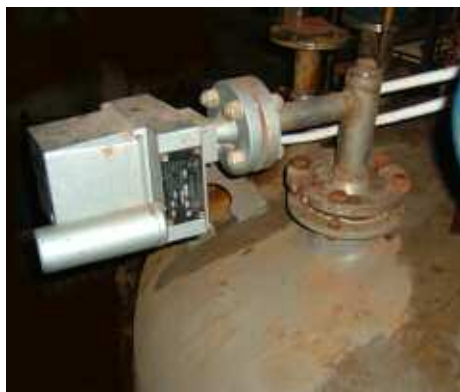
Soviet torque tube displacer transmitter.
