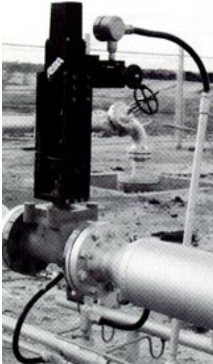
This solar powered electrohydraulic Valve actuator develops 4,000-lb. of thrust and is used to control flow through a remote Venezuelan oil pipeline. (Rexa)
