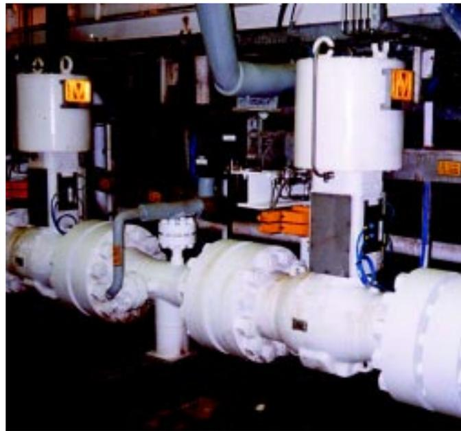
**D**ue to environmental constraints and cost saving, HIPPS has gained popularity over the last years as the last line of defence, replacing pressure safety valves (PSV), blow down and flare systems. Although HIPPS is applied for more than a quarter of a century, design and implementation of HIPPS is still not as obvious as one might expect. The main reason for this is the way the IEC 61508 and the more recently introduced IEC61511 standards are written.
