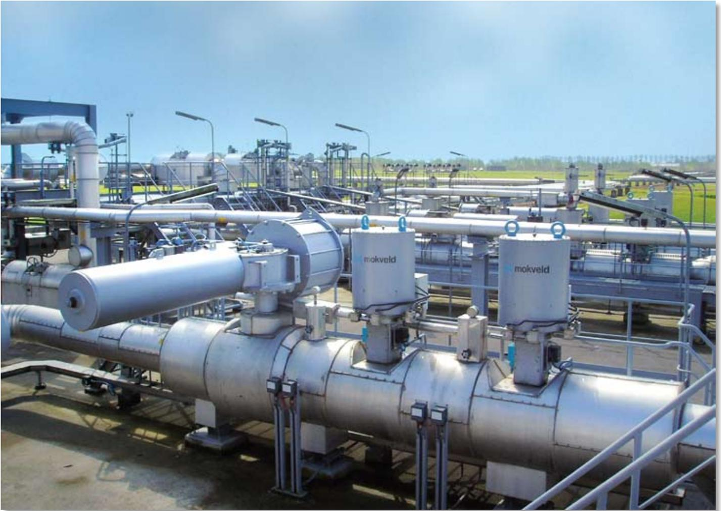
Fig. 2. One ball valve for ESD and two axial on-off valves for HIPPS. (The Netherlands)
