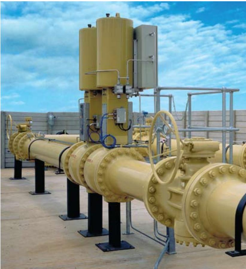
Fig. 3. A typical control and safety system consisting of an axial control valve and an axial on-off valve (HIPPS valve) according to IEC 61508. (South Africa).
