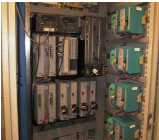
Figures 1 & 2: Yokogawa DCS & ASI master gateways & power supplies, 4 FF I/O cards
