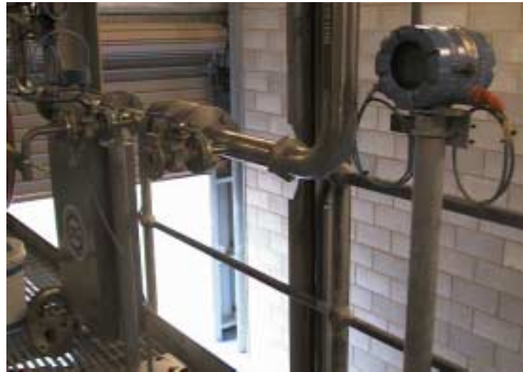
Figures 3 & 4: Mass & mag flowmeters (Fisher Rosemount) used in conjunction with Valtek / Somas Control valves.
