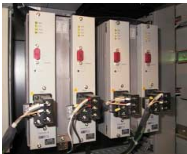
Figures 1 & 2: Yokogawa DCS & ASI master gateways & power supplies, 4 FF I/O cards
