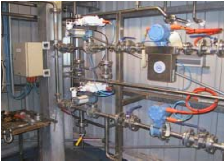
Figures 3 & 4: Mass & mag flowmeters (Fisher Rosemount) used in conjunction with Valtek / Somas Control valves.
