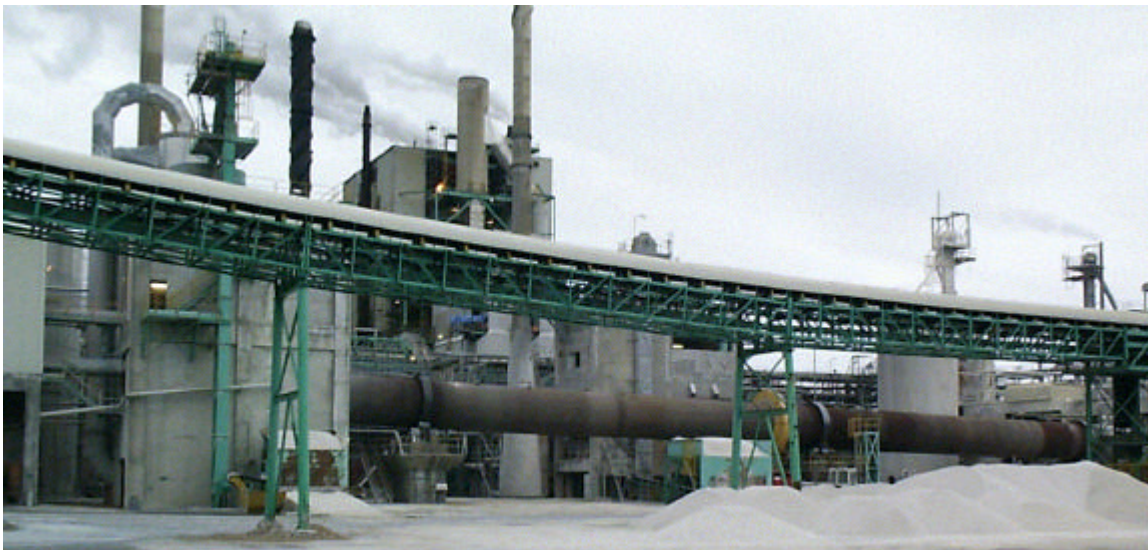
Figure 8 CHH Tasman pulp mill, limekiln
