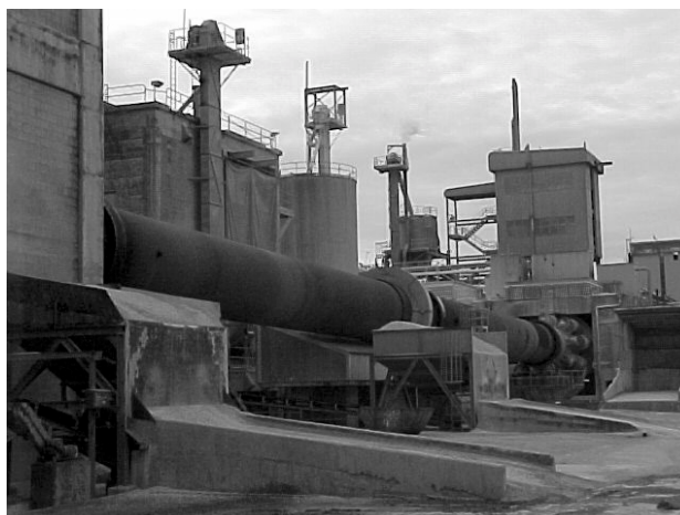
Figure 2 - View of Lime Kiln No.2
