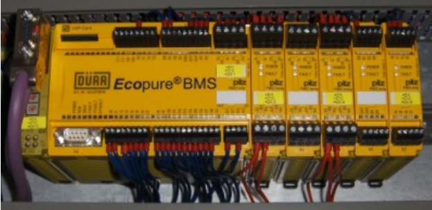
Fig. 1 The PNOZmulti safety system saves space in the control cabinet.
